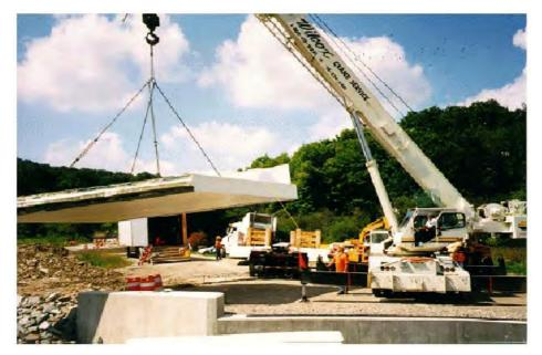
Figure 4 – New modular FRP bridge deck (Source [20])
