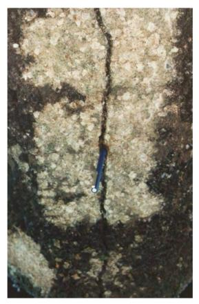
Figure 9 – Typical longitudinal crack in concrete due to alkali / silica reaction (Source [23])
