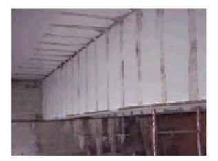
Figure 5 – Externally bonded FRP plates (Source [21])
