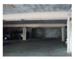
Figure 1 – Strengthening / stiffening suspended concrete slab with steel beams
