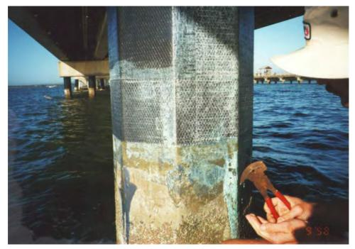
Figure 10 – Externally bonded CFRP (Source [23])
