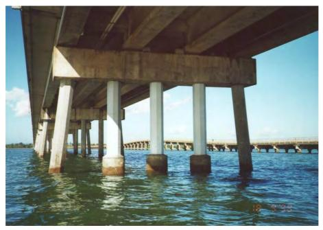
Figure 8 – Houghton Highway substructure Source [23])
