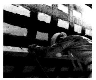
Figure 7 – CFRP strips located on PC shell (Source [18])
