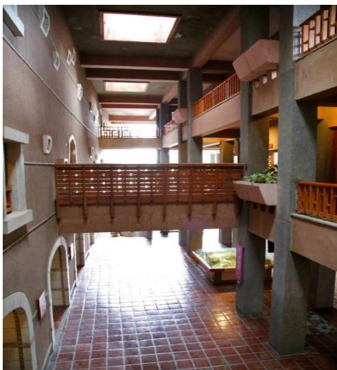
Figure 14: Skylights above corridor
