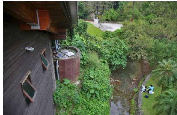
Figure 8: Rainwater storage
