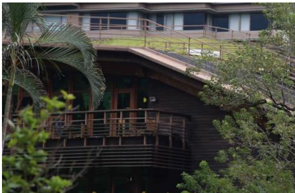
Figure 7: Roof solar panels and roof soil layer
