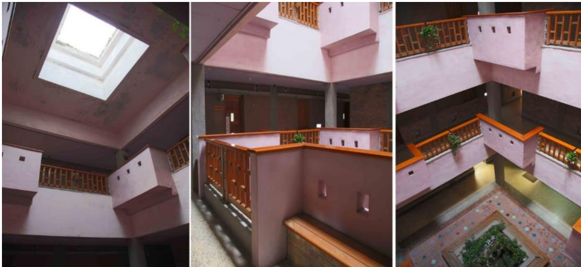
Figure 13: A skylight at roof forms a small courtyard on the ground floor
