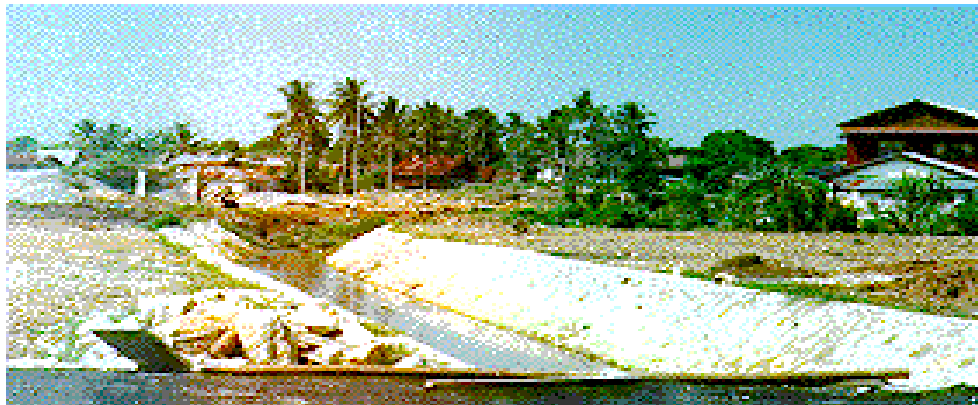
Figure 1 : Main Drain from Teluk Kumbar New Township Discharging into Existing Earth Stream
