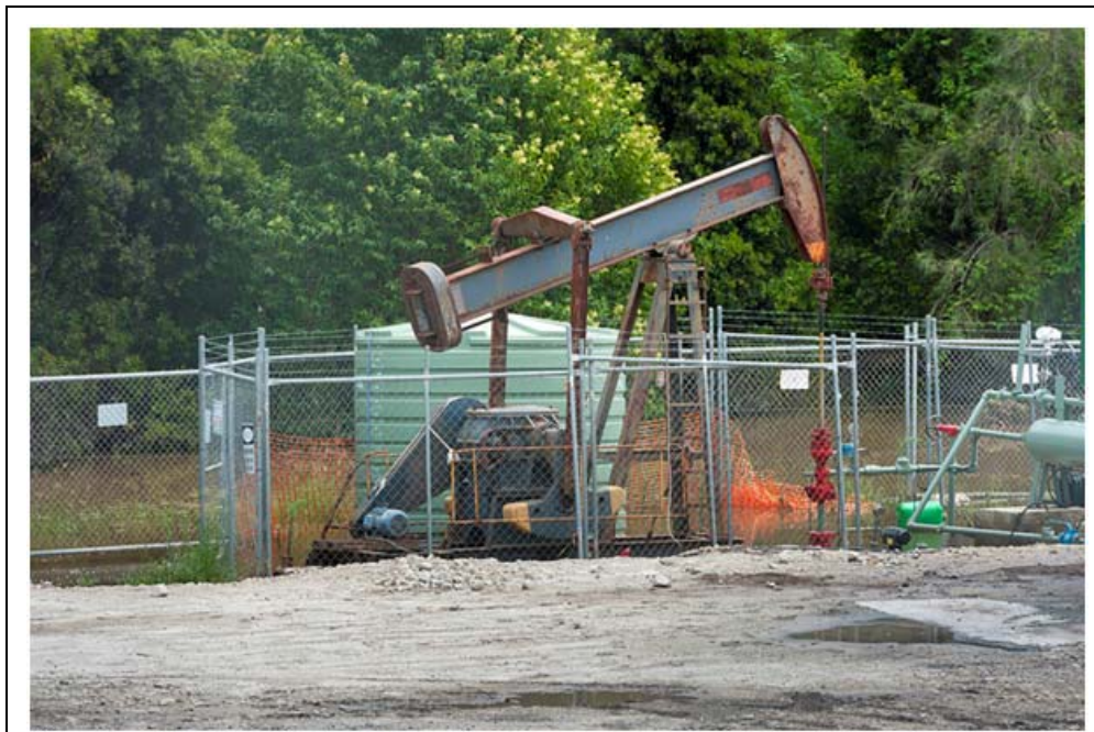
Figure 1 CSG Well at Menangle showing wellhead within fenced area
