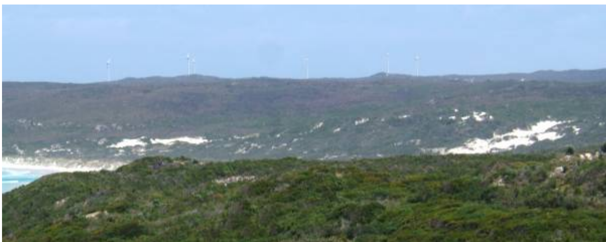
Ten Mile Lagoon Wind Farm
