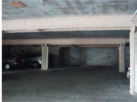
**Figure 1 – Strengthening / stiffening suspended concrete slab with steel beams**
