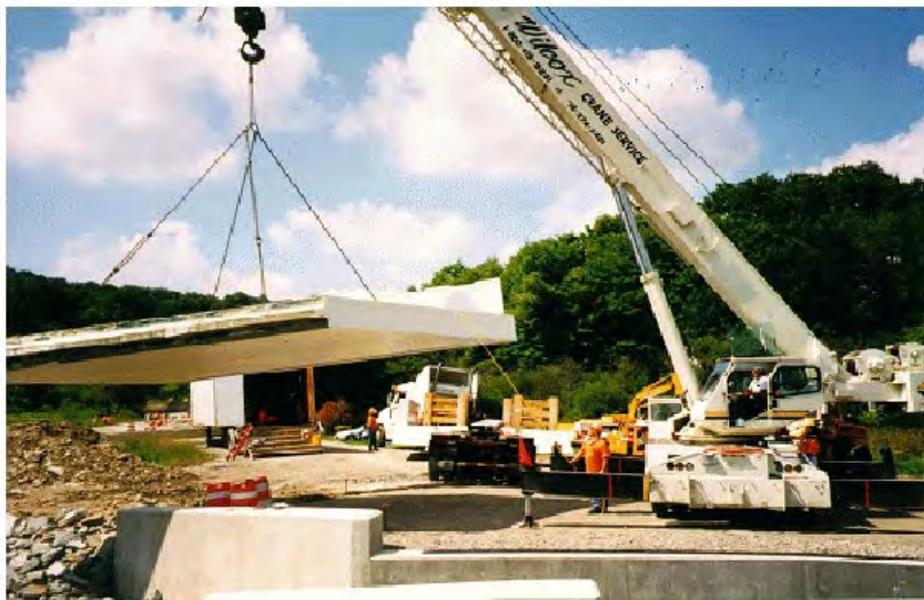
**Figure 4 – New modular FRP bridge deck
