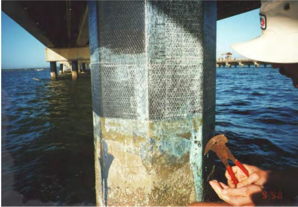
**Figure 10 – Externally bonded CFRP
