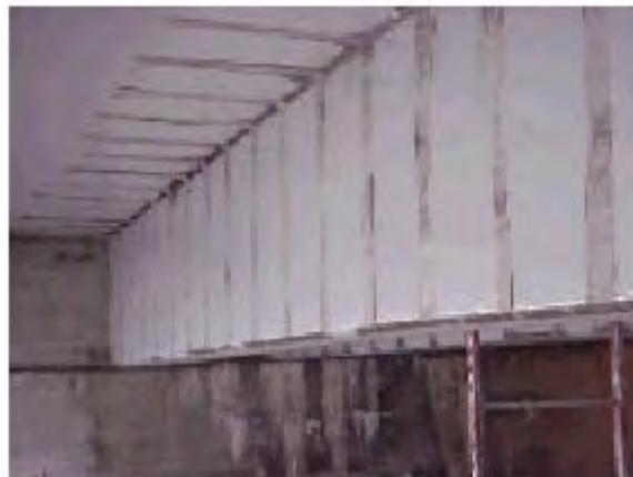
**Figure 5 – Externally bonded FRP plates
