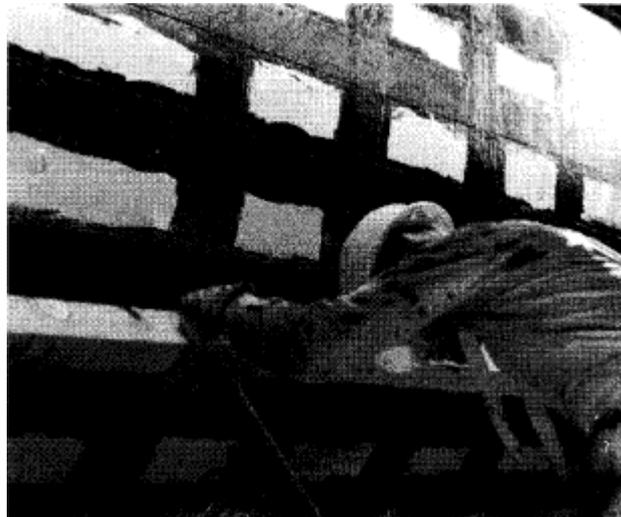
**Figure 7 – CFRP strips located on PC shell**
